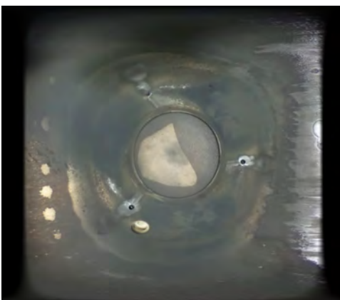
Combustion Chamber Indicating underside of Cylinder Head , Exhaust Valve , Injectors Tips
